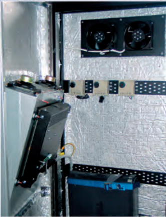
Demonstration of the Climate Control Unit in the outdoor Hawk
